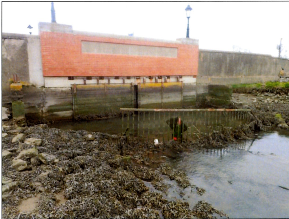
Plate 4.5 Section 10; the tidal sluice at Portmarnock Bridge
