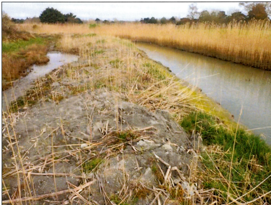
Plate 4.6 Section 10; the spoil from a recent dredging operation
